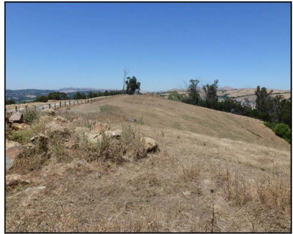
Figure 5b. Looking north
